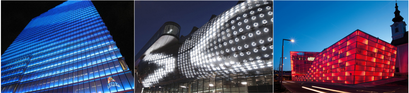
Figure 1. Light emitting media façades embedded into contemporary architecture that may display interactive content (from left): Dexia Tower, Brussels, Belgium (Photograph by Eddie Janssens), Kunsthhaus, Graz, Austria (Photograph by Nicolas Lackner) and the ARS Electronica Center in Linz, Austria (Photograph by Nicolas Ferrando & Lois Lammerhuber).
